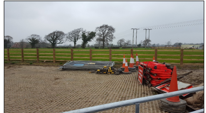
Plate 7: View of eastern part of Site, looking north
